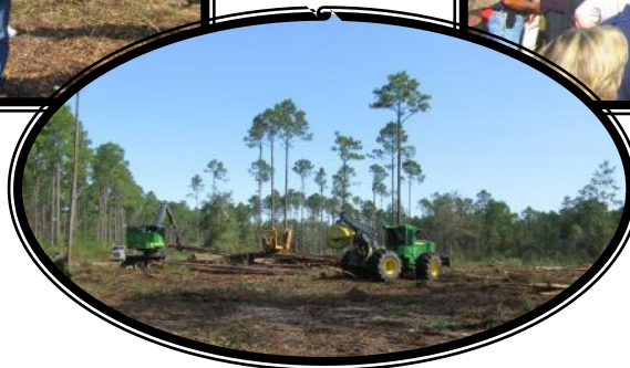
K & B Land & Timber jobsite
